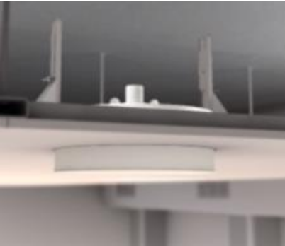
Through the ceiling
