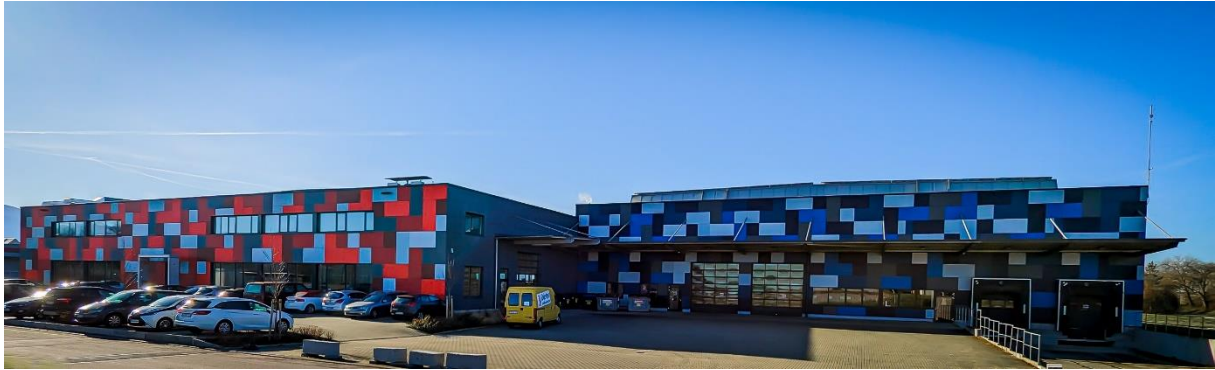
Exterior view of the production hall and warehouse in Heitersheim, Germany
